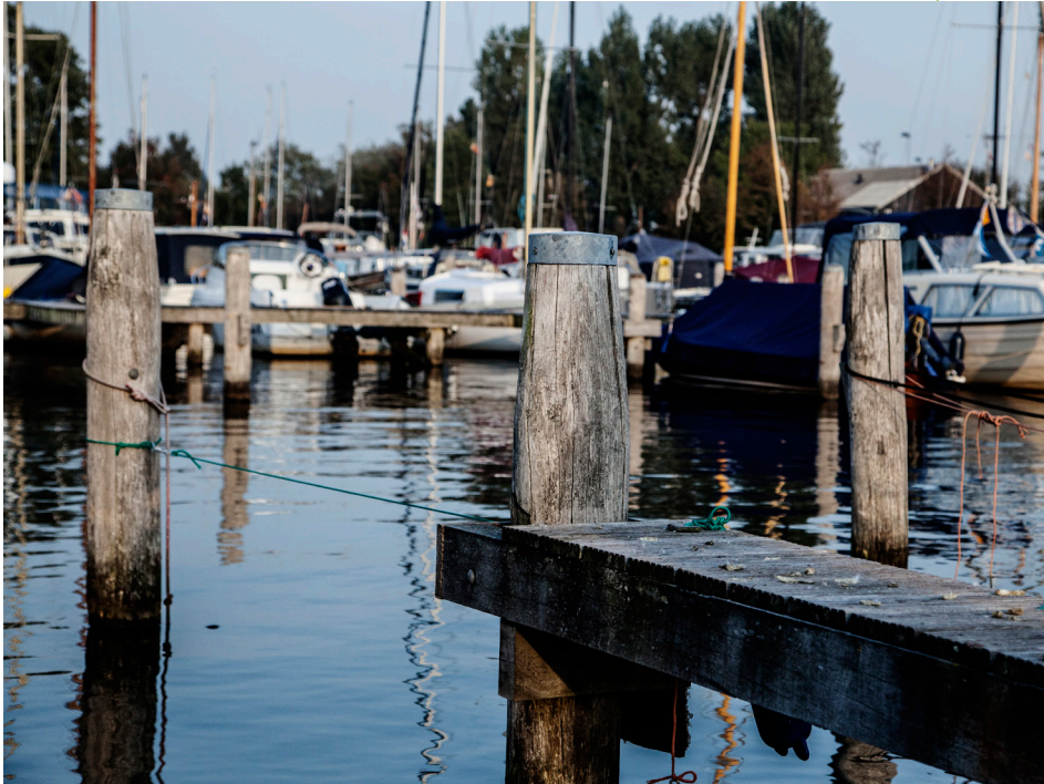
Manbarklak round poles in Akkrum Marina from 2009 and still in good condition. (Photo: Mark van Benthem - Probos)
